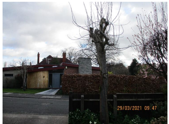
No. 2 Winchester Avenue as viewed from site.
