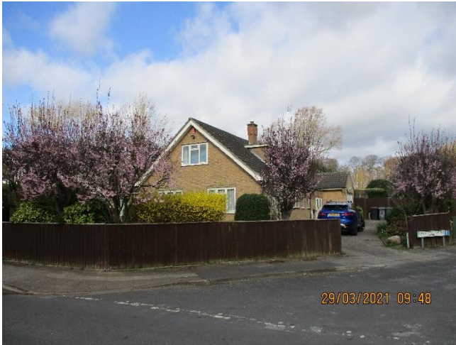
Front (SE) and side (NE) elevations.
